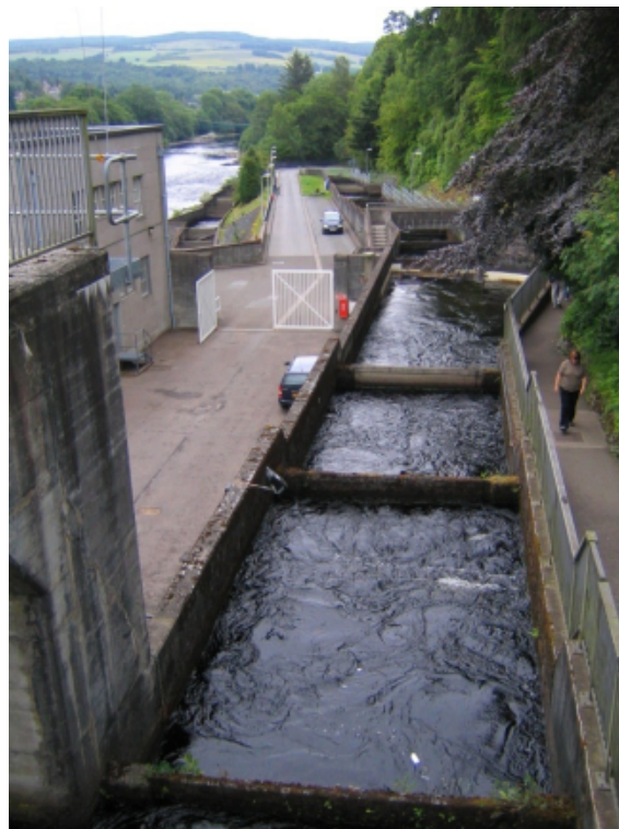
Figure 3.11: Pool-type fish pass, Pitlochry Dam and hydropower station, River Tummel, Scotland (Photo: Marq Redeker)
