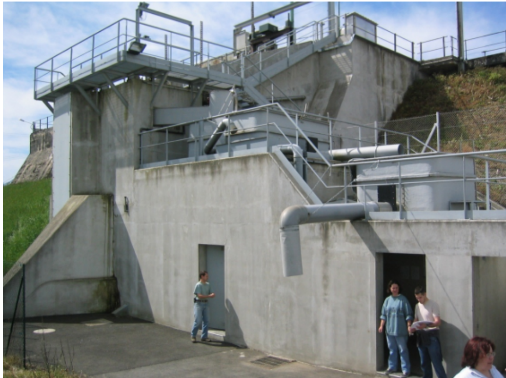
Figure 3.15: Trapping station for downstream migrating salmon smolts in Camon, Garonne River, France (Photo: Marq Redeker)
