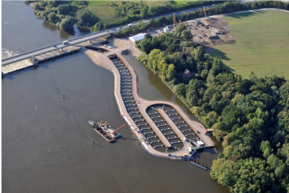
Figure 3.10: Vertical slot fish pass Geesthacht, Elbe River, Germany (Photo: Vattenfall)
