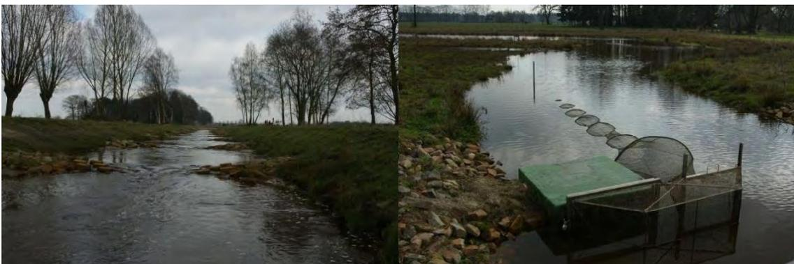
Figure 19. The shallow V notch pass Kawaise Loop (left, 12-03) and the upstream inlet of the fish siphon pass with fish trap and coupling piece (right, 12-03)
