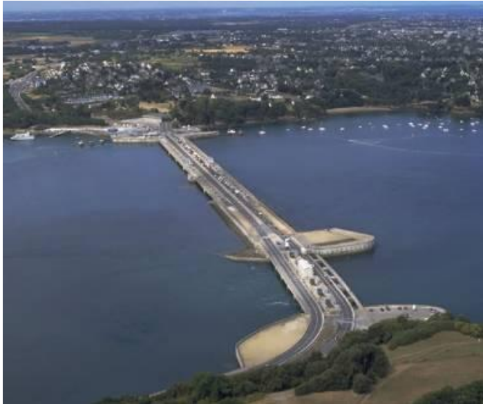
Figure 2.1: La Rance tidal barrage, France.
