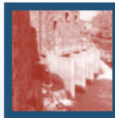
Powerhouse dressed in local material © IT Power
