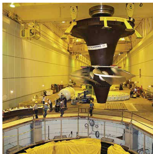
Figure 3. Voith Hydro Minimum Gap Runner (MGR) during installation at Wanapum Dam on the Columbia River in Washington State in 2005. Photo credit: Grant County Public Utility District.
