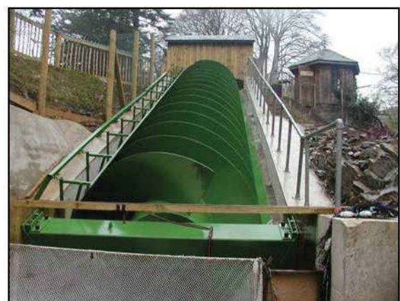
Figure 4. Archimedes screw turbine installed on the River Dart in the UK. Photo credit: Fishtek Consulting.
