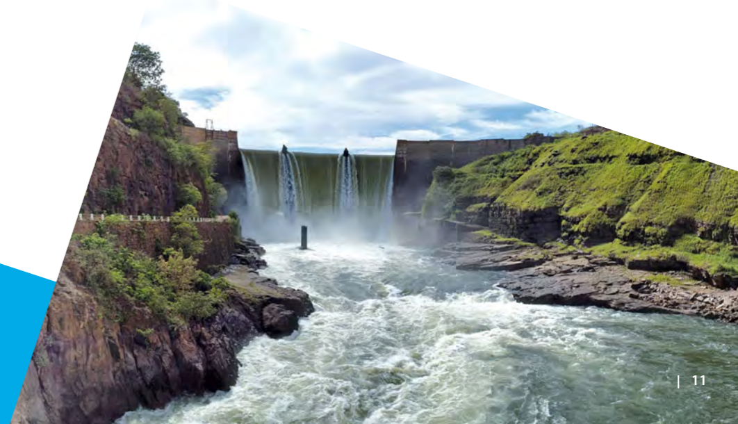
The Cambambe power station in Angola. Credit: Voith Hydro.
