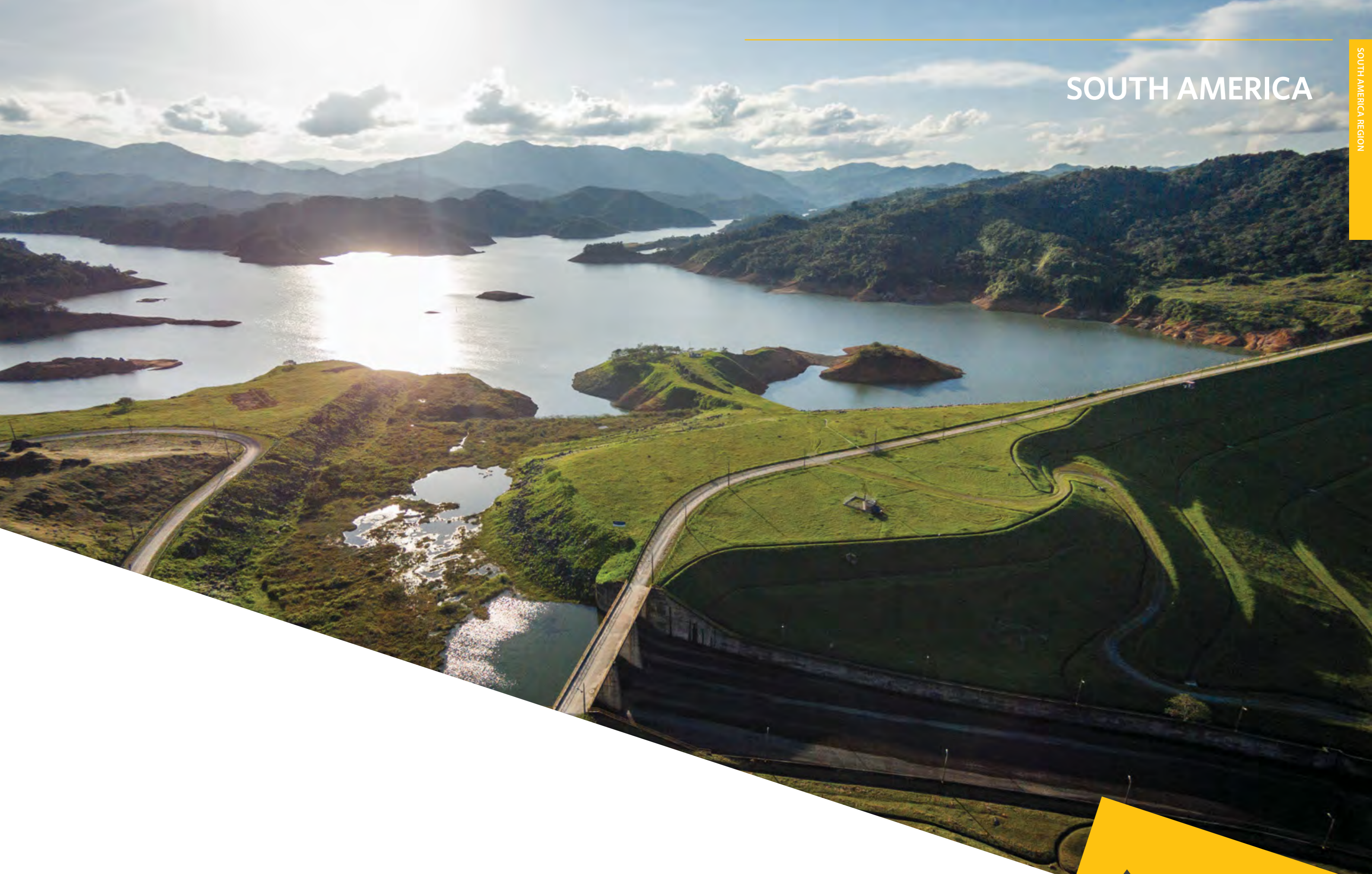
▲ The Jaguas hydroelectric power plant, Colombia. Credit: Isagen S.A. E.S.P.
