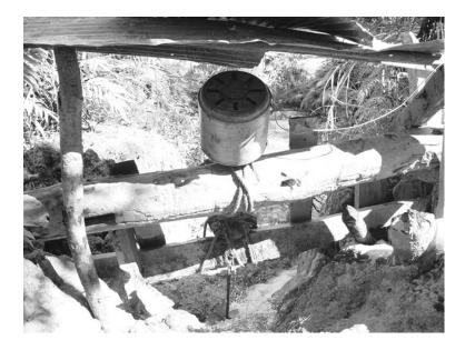
Fig. 3 Modified propeller Pico Hydro system in Thapene village.
