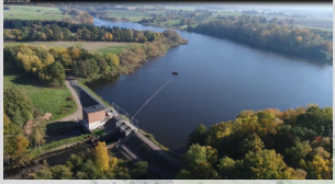
Pre restoration conditions, HPP1
