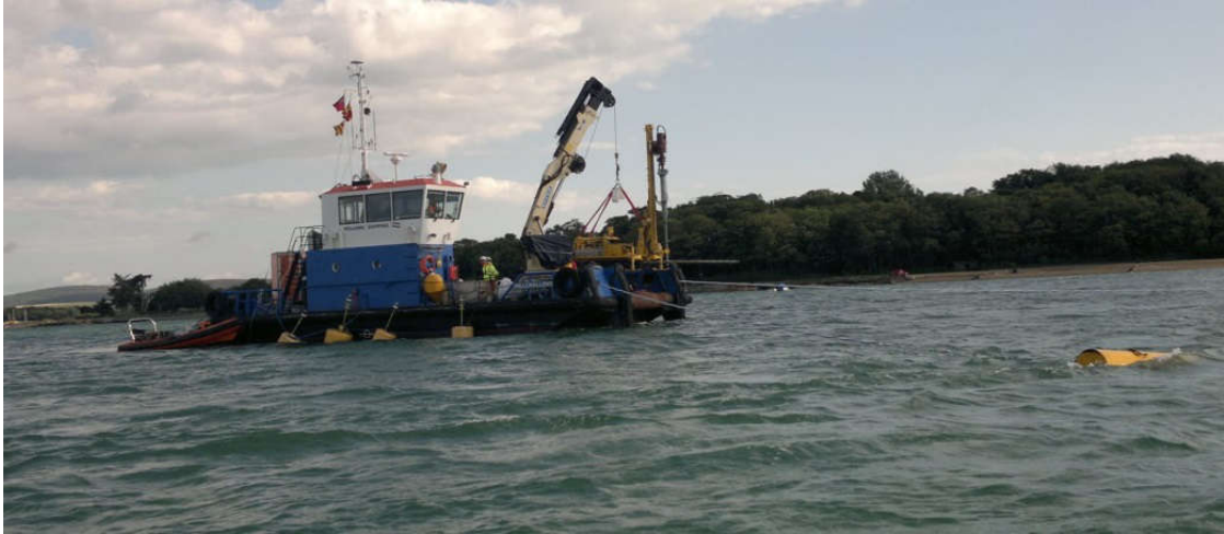
Figure 2 Willchallenge deploying the drill rig on the 20 th August 2014.
