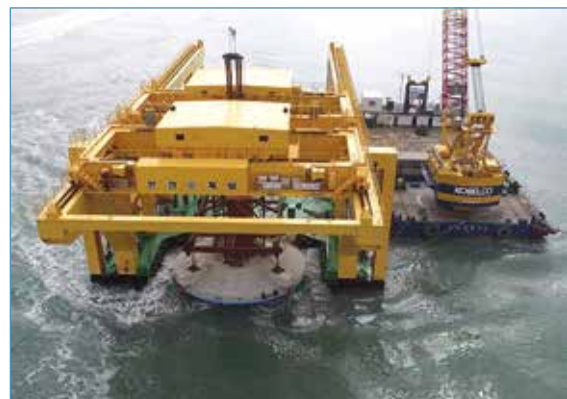
200 kW active-controlled tidal energy converter in fabrication and installation of its substructure
