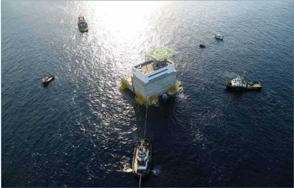
Installation of PLOCAN offshore platform
