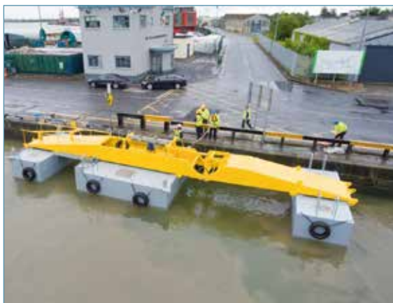
SeaPower Platform at Foynes Port, Co. Limerick in 2016
