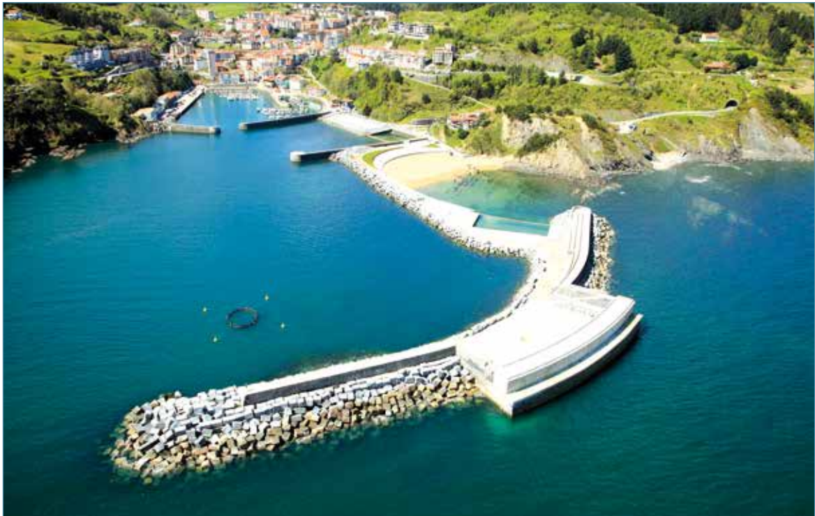
Mutriku wave power plant
