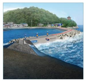
WEC applicable to breakwaters on remote island
