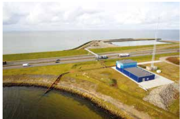
Redstack pilot facility
