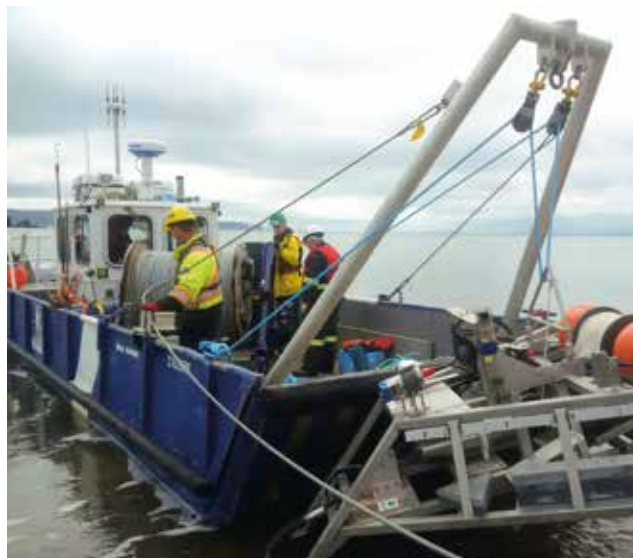
Installation of FAST platform, photo credit: FORCE
