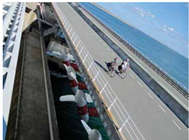
Tocado tidal power plant in the Eastern Scheldt (Photo credit: Tocardo Tidal Power)
