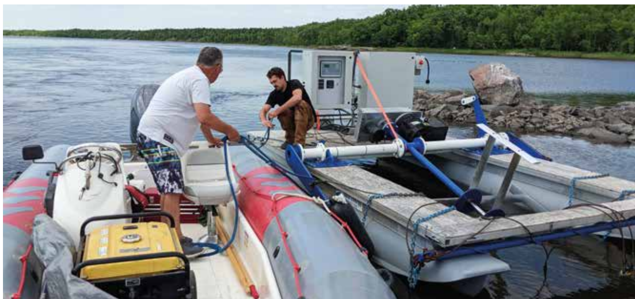
Installation of the New Energy Corp. Turbine, photo credit: CHTTC
