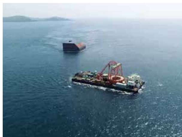
Installation of offshore cables nearby the existing OWC WEC
