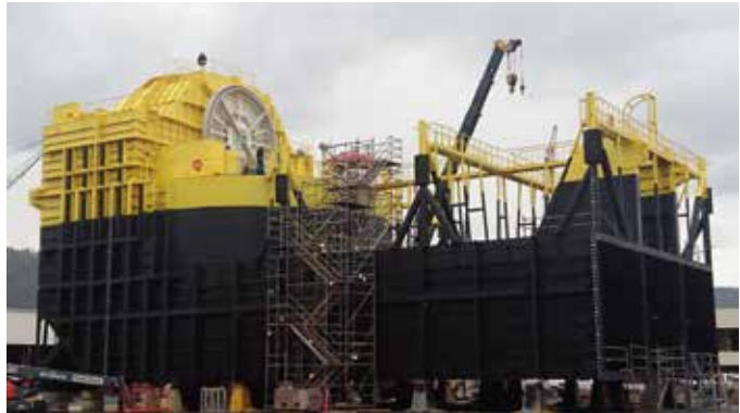
OE Buoy Build December 2018
