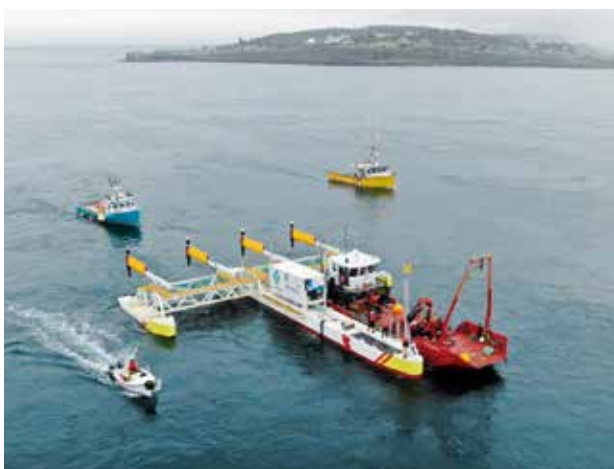
PLAT-I platform being connected to the moorings on September 18th, 2018 (source: SCHOTTEL HYDRO)
