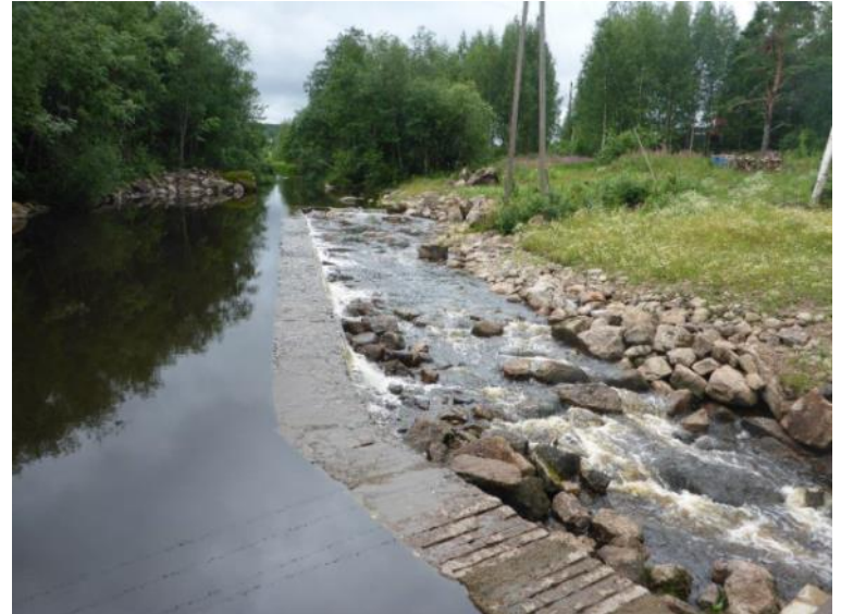
From the dam site towards upstream
