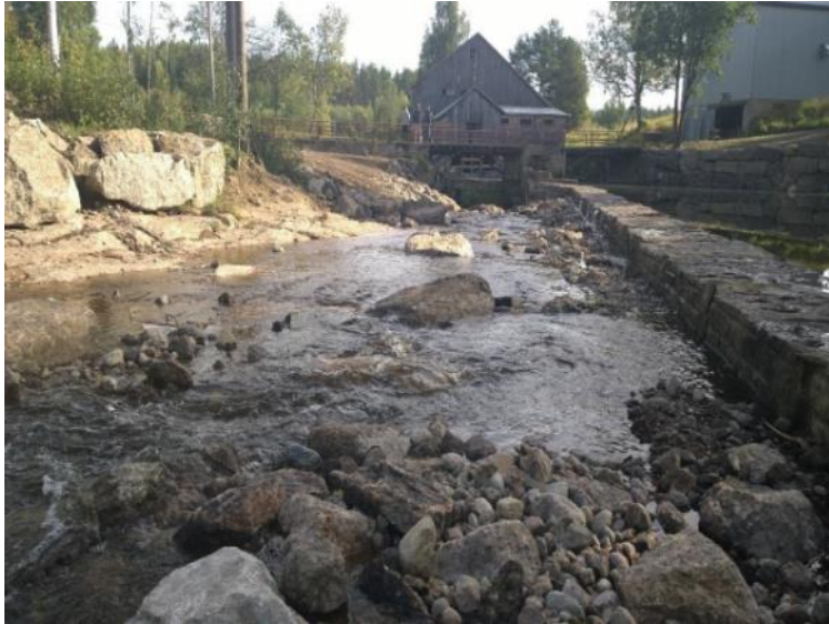
Towards the former dam site downstream
